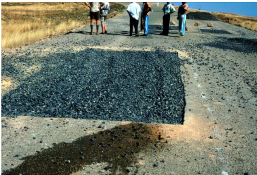
Fig. 4. Road works straddling the road without signs or attendants.
